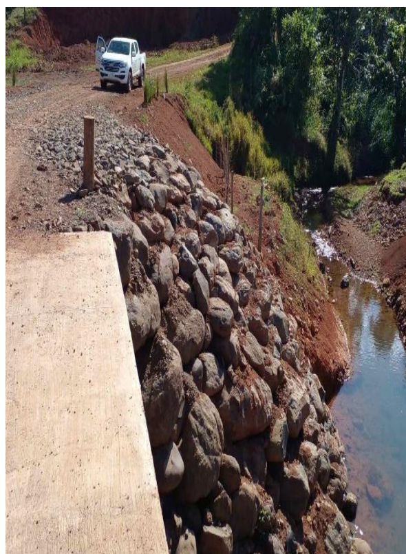
A bridge in Waiqe Sector after repair
